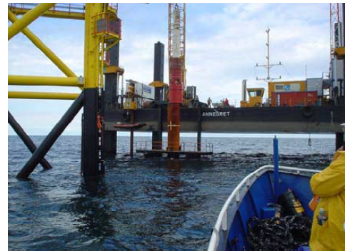
Fig. 4: Pile driving FINO 1 (jacket, working platform, pile hammer helmet)
