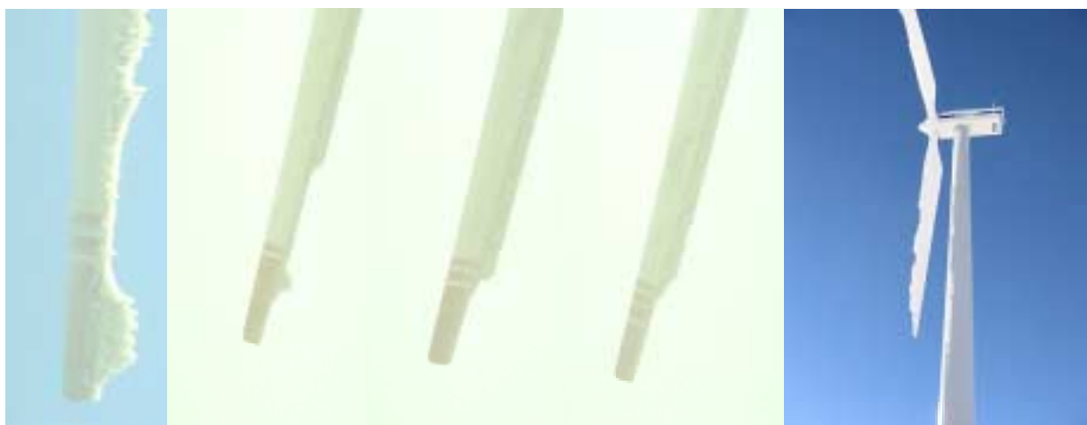
Figure 8 Leading edge ice accretion during idling (left side), unsymmetrical icing at a 3-bladed rotor during operation (middle) and saw blade-like ice accretion (right side).
