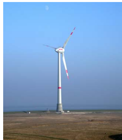
Fig. 3: Enercon E-112 on the DEWI-OCC test site at Cuxhaven
