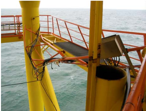
Pict. 1, right: Lower working platform in August 2006 Pict. 2 and 3, below: damage caused by the storm of 1 November 2006. Several floor gratings had been torn from their mountings, and parts of the railings showed heavy deformation.
