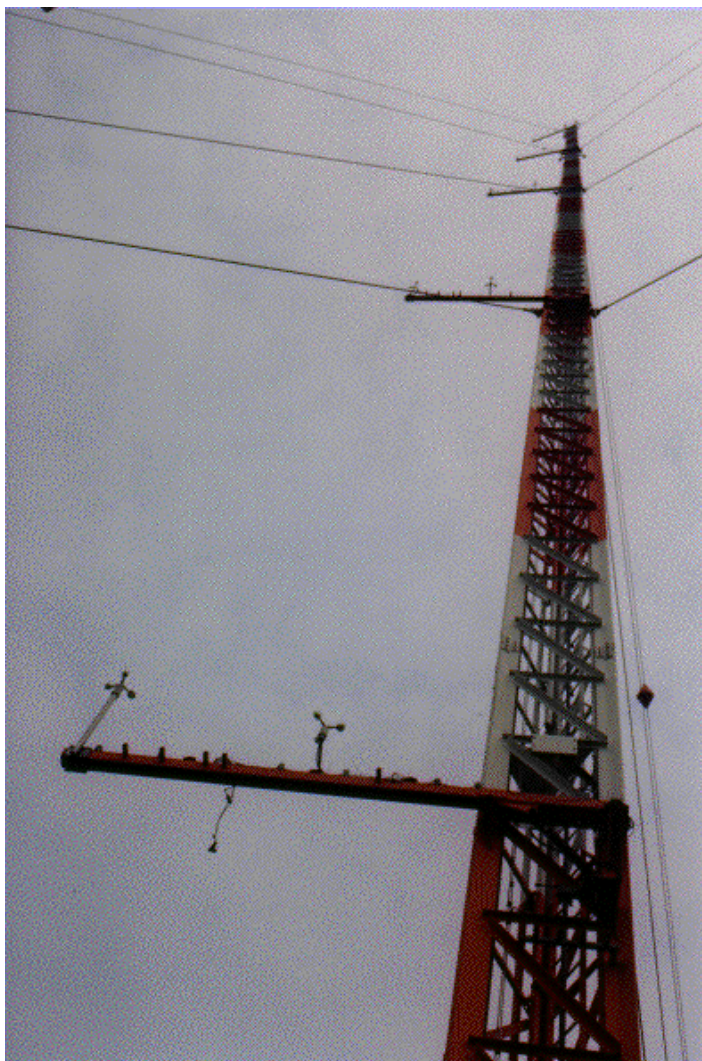
Abb. 1: 130 m Meßmast des DEWI Abb. 1: 130 m wind measurement mast of DEWI
