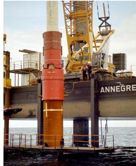
Fig. 1: Hydraulic hammer on a pile of FINO1.
