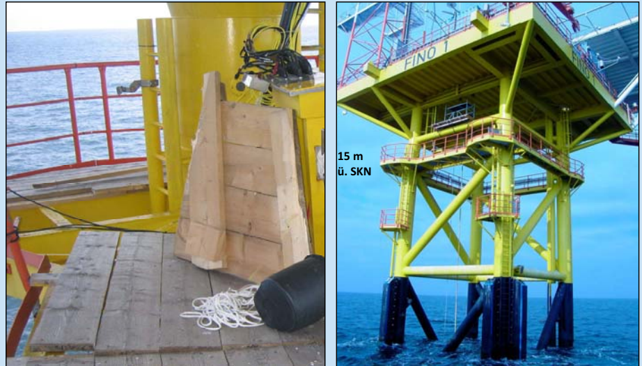
Fig. 1: On 9 November 2007, broken wooden planks on the working platform 15 m above chart datum (left). Basement of the FINO 1 research platform and location of the working platform.
