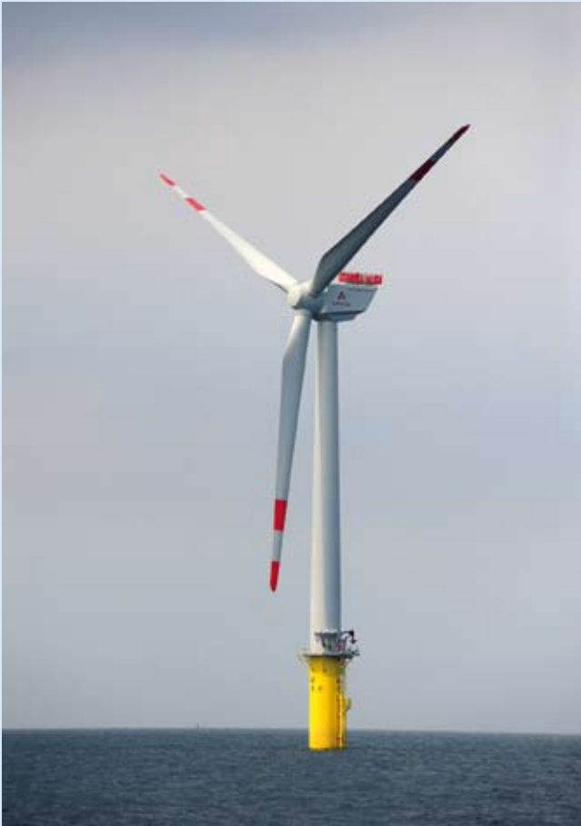
Fig. 1: The first wind turbine in the alpha ventus offshore test site (Source: DOTI 2009)
