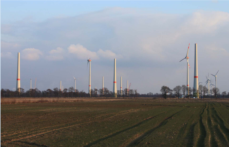
Fig. 4: Citizen-owned Saterland wind farm realized as a repowering project in 2013
