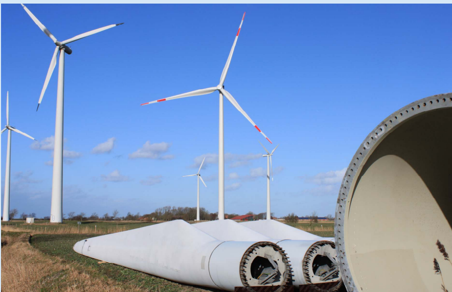
Fig. 5: Repowering 2013/14 in the Bassens wind farm: A modern wind turbine with 3 MW (in the center) has the same capacity as five old wind turbines with 600 kW
