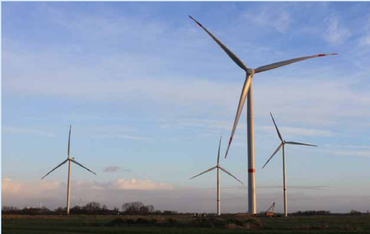
Fig. 5: The new test site at Anzetal near Wilhelmshaven was also classified as a repowering project according to the BNetzA register (photo: Bernd Neddermann)
